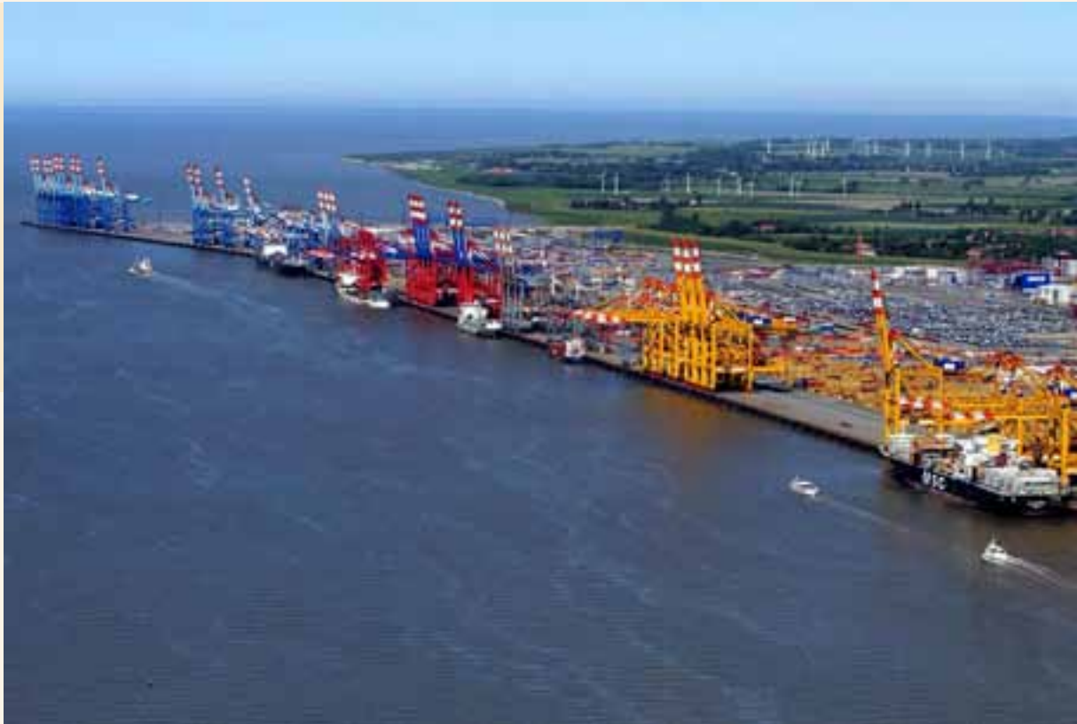
Containerterminal in Bremerhaven
